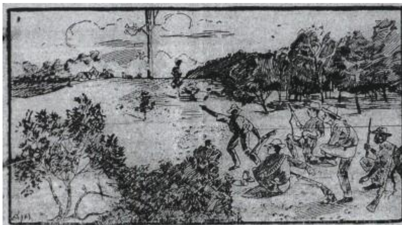
Scene of the Kenniff arrest Near the Maranoa River just south of Mitchell, as depicted in a contemporary newspaper report. Note the police officers removing their boots in an unsuccessful attempt to sneak up on the Kenniffs. sketch from Sunday Truth newspaper, 6 July 1902
